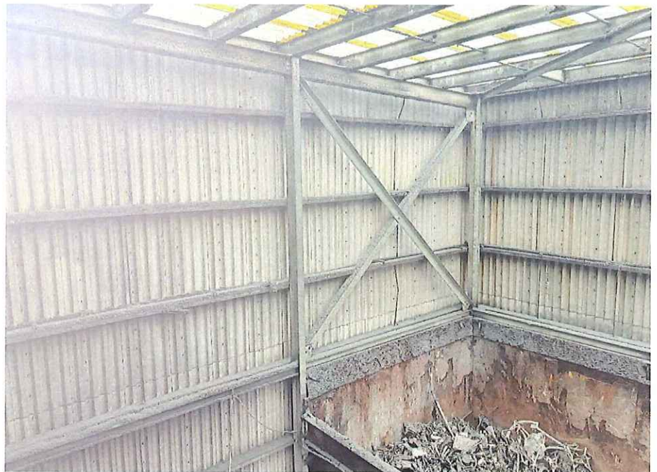
Ash Building Refurbishment
