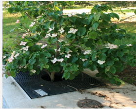
Tree box filter in East Lyme, CT
