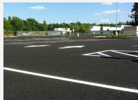
Pervious asphalt at Goodwin College
