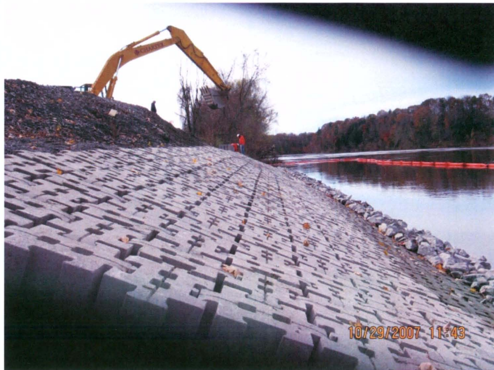
Figure 3. Articulating Blocks being Placed at Stream bank Restoration Project in New Hampshire.
