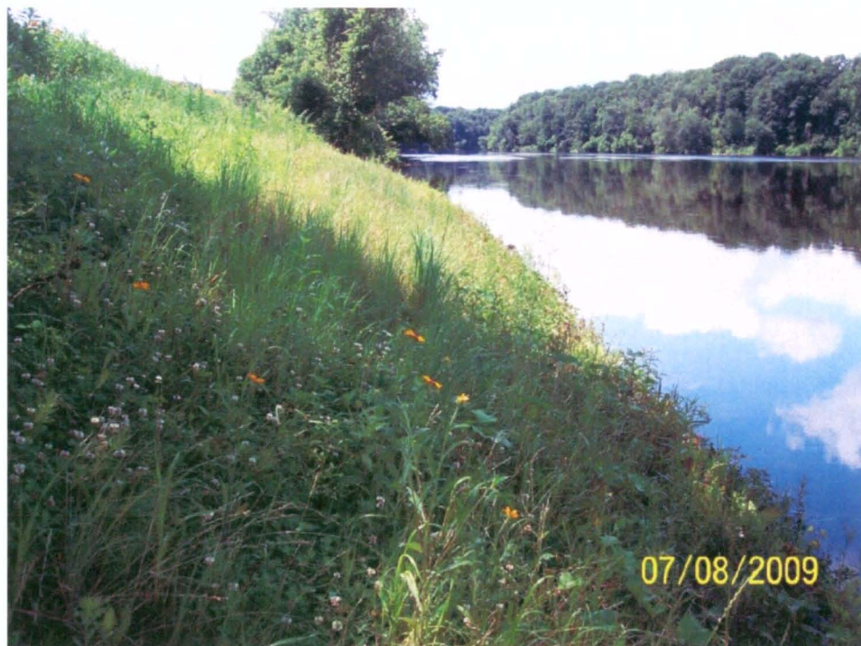
Figure 4. Photo of Completed New Hampshire Project with Re-vegetation.
