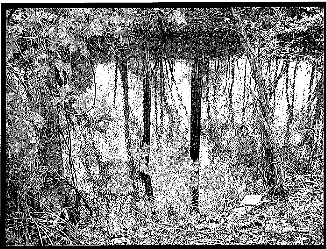
PHOTO 4 Two wooden piers along east side of brook.
