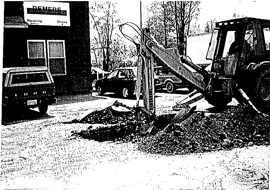
Photograph 1: Suspect UST Area 1, Test Pit Excavation
