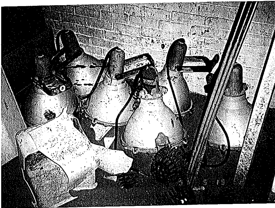
Photograph 13: Mercury Vapor Lights Within Room #1C
