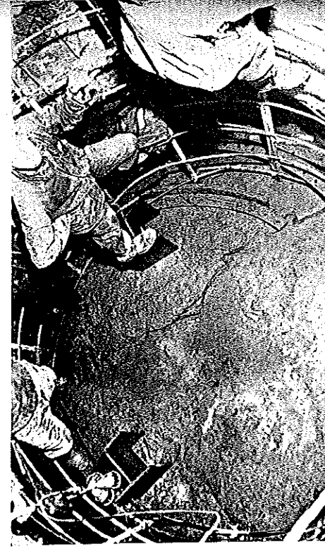
SAND-HOGS REACH BED-ROCK. Under air pressure of 45-47 lbs., they were allowed to work only \frac{3}{4} of an hour, spend \frac{1}{4} of an hour decompressing, and rest five hours before working again.
