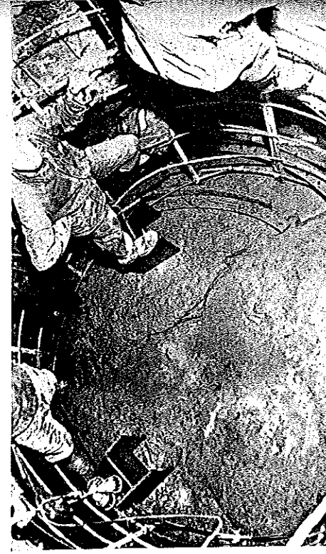
SAND-HOGS REACH BED-ROCK. Under air pressure of 45-47 lbs., they were allowed to work only \frac{3}{4} of an hour, spend \frac{1}{4} of an hour decompressing, and rest five hours before working again.
